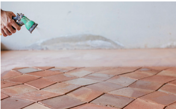
Wetting of pieces prior to grouting
