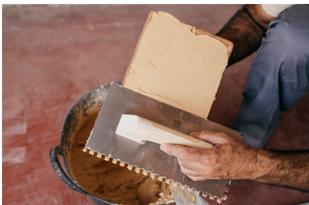
Adhesive layer application on the back of the tile
