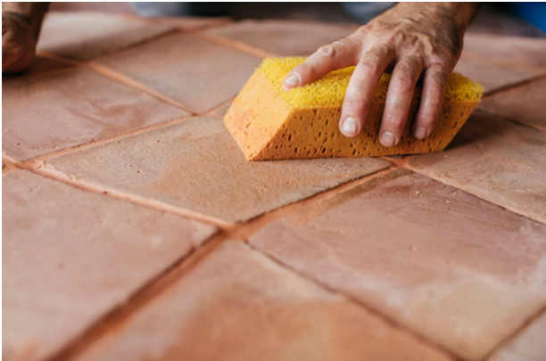
Cleaning grouting material with a sponge
