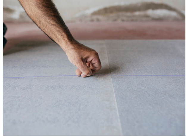
Stakeout of laying lines with tracer
