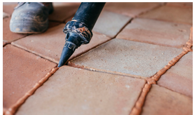
Joint sealing with grouting material
