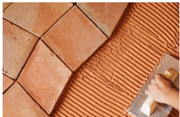
Adhesive combed with notched trowel on support
